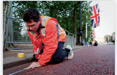
Laying Out a Calibration Course
